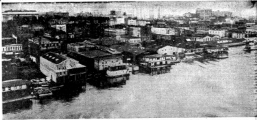
EARLY VIEW — Picture to right shows what west bank of Willamette River looked like in about 1910, before Madison and Taylor streets were built. Harbor Drive was built. Picture below it shows construction of drive in 1943, looking north from about SW Water Street.
