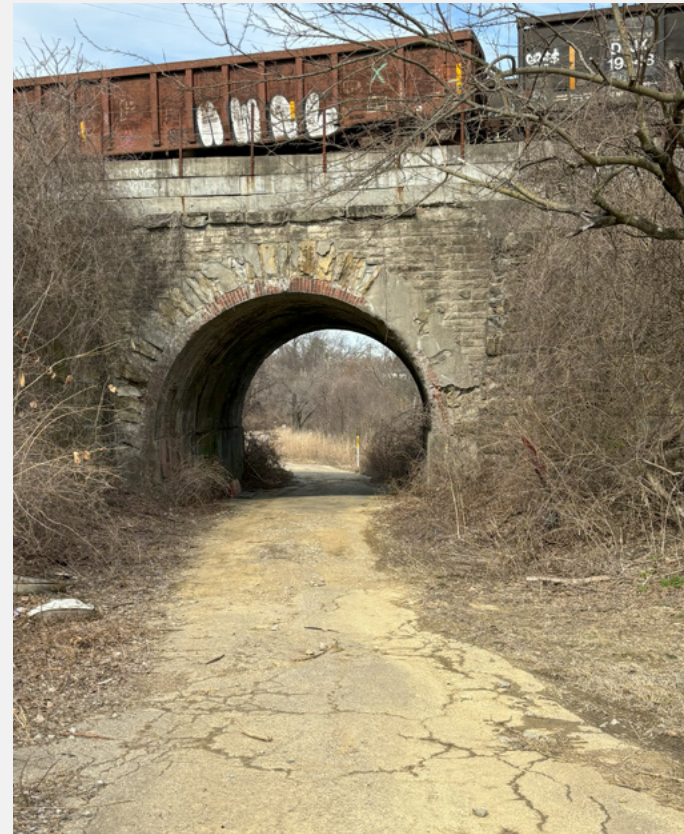
EXISTING HARRIS AVE TUNNEL
