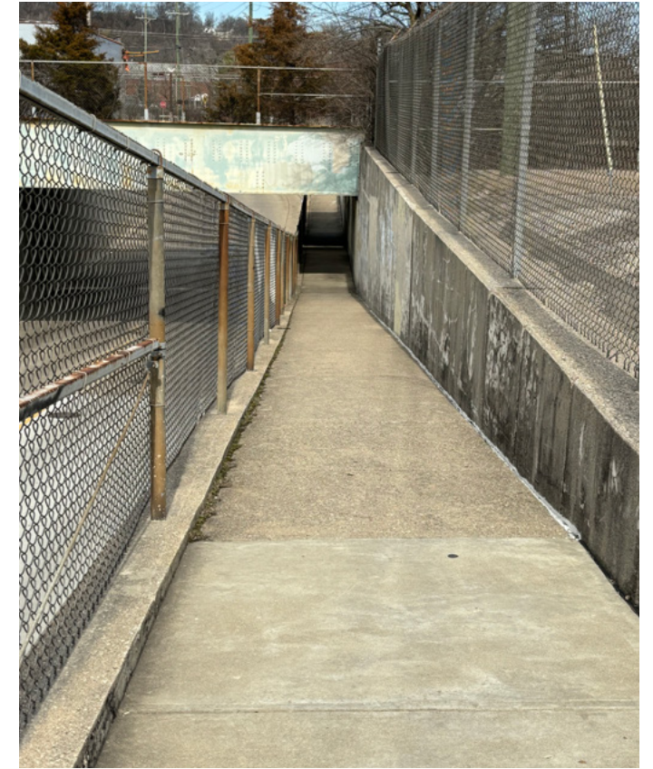
28 Forest Ave Railroad crossing
