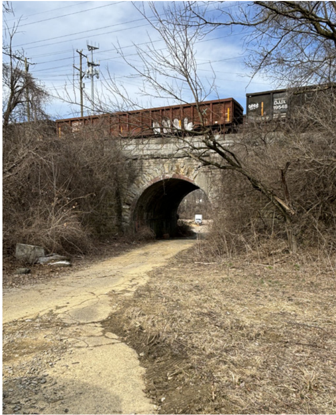
2 Harris Ave tunnel
