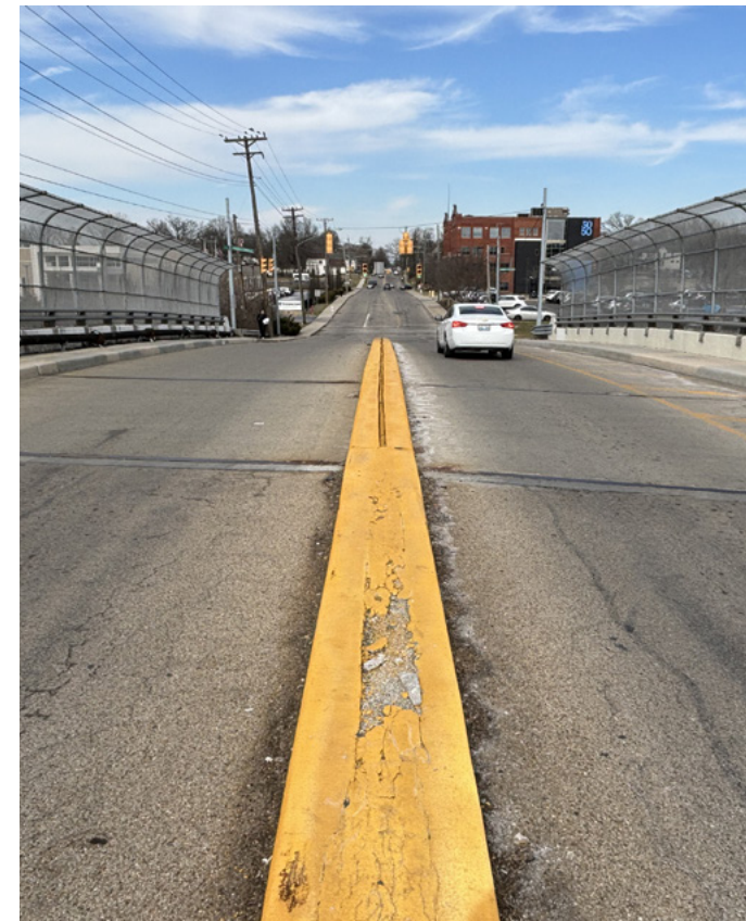
21 Section Ave bridge
